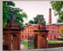
Gateway, caretaker's lodge
